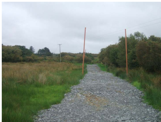
Figure 5.2 Temporary Stone Road
