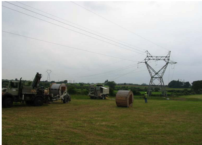
Figure 5.8 Typical Stringing Equipment
