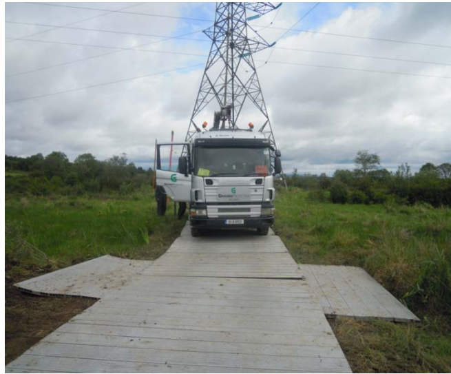
Figure 5.1 Temporary Aluminium Panel Tracks
