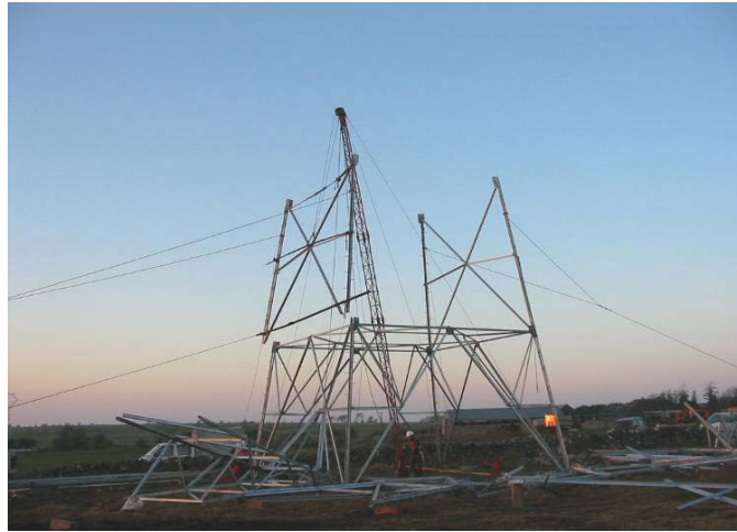
Figure 5.5 Derrick Pole at Tower Base
