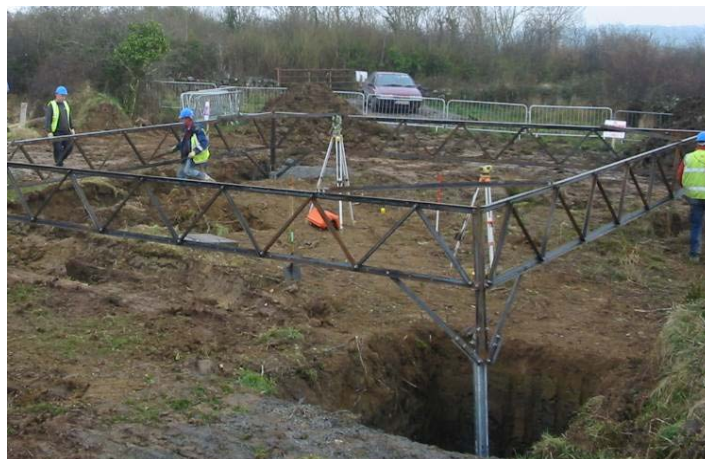
Figure 5.3 Setting Template being prepared for Final Concreting
